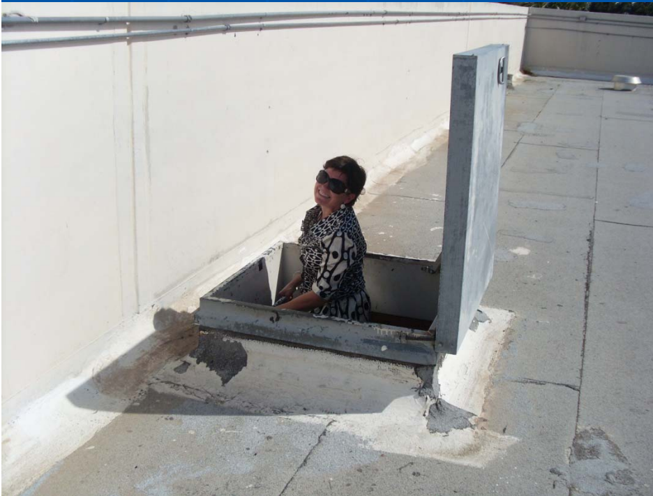
Danger! Access and Climb
