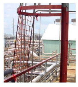
**Step 1.** Center the CageX Net over the ladder cage support and fasten with one chinch strap at the center as shown with the letter "A". Spread the net along the cage support and attach the left and right corners as shown with chinch straps. Spread the net along the hand rail and install two chinch straps at the left and right corners. Attach the last chinch strap at the bottom center and secure it to the hand rail.
