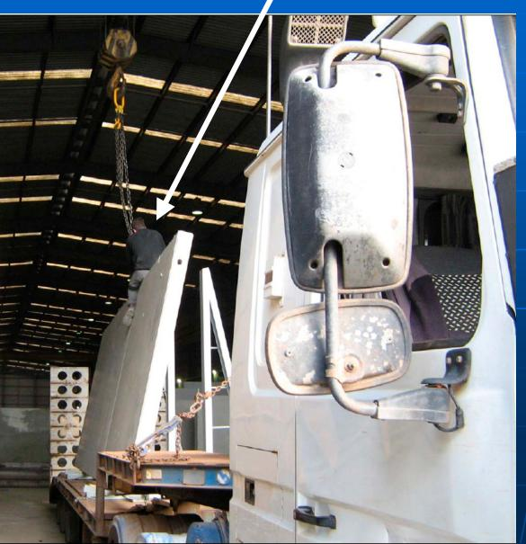
Climbing the load to detach a chain hoist
